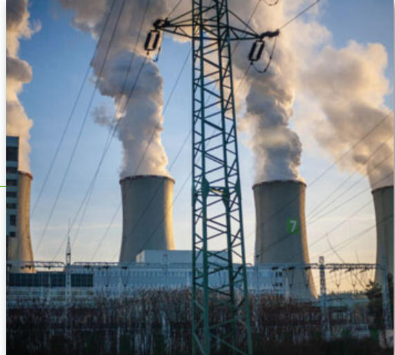
Chvaletice coal-fired power plant. Photo: Laura Otýpková
